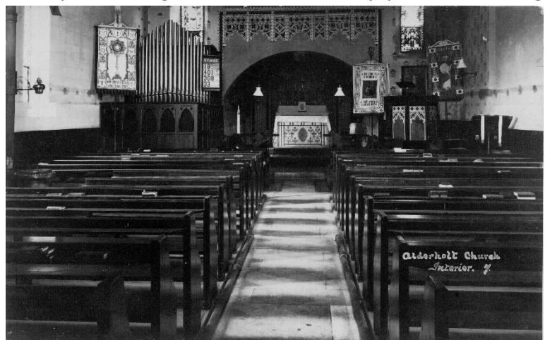
The interior of the church before the new nave was added.
