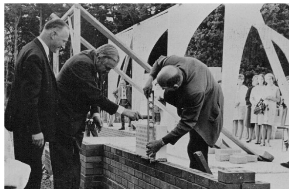
New Hall Stone Laying in 1967
