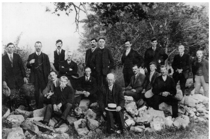
Parishioners collecting stones for the new Chancel.
