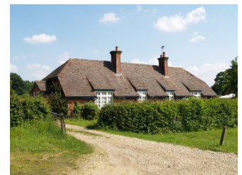
A typical Cranborne Estate semi-detached bungalow
